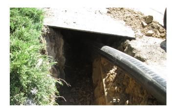
New 16 inch pipe being installed by pipe bursting.
